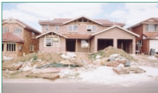
Fines issued to this site were for general untidiness of the site, the positioning of the stockpile, the need for maintenance of the sediment fence and the lack of an all weather access point.
