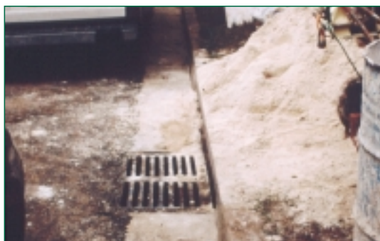
Soil in street gutters are a clear sign of inadequate erosion and sediment controls. A sediment fence and grass filter strip could assist in this situation, stopping the dirt before it enters the stormwater system.
